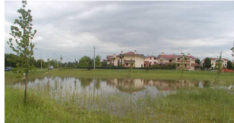
PROTOTYPE STORM WATER MANAGEMENT FACILITY
